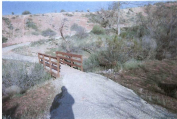
This is a 6'x18' wood foot bridge on the hiking trail.
