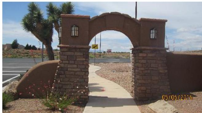
Brick and stucco walls around the entry ways may need to be repaired or replaced at some point. We have budgeted for this in 2033.
